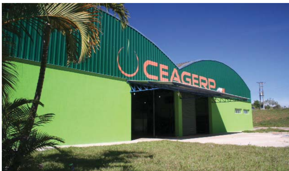
Fachada principal da Ceagerp
